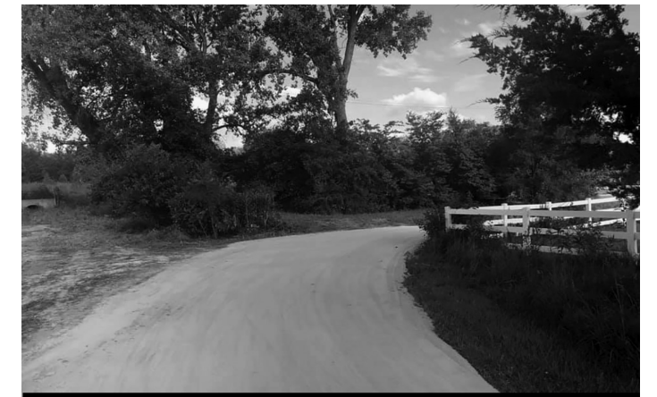
Repaired corner on the MoPac Trail at A Street and 98 Street
