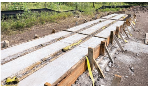
Unsealed concrete castings for the concrete bridge deck.
