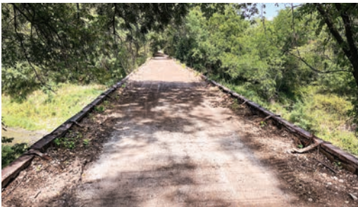
The former railroad bridge, cleared of vegetation debris.
