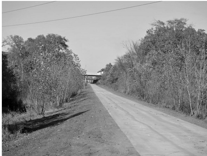
The newly constructed North Jamaica trail looking north from the Salt Creek Levee trail junction.
